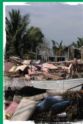
Tsunami damage, 2004 Indonesia.
